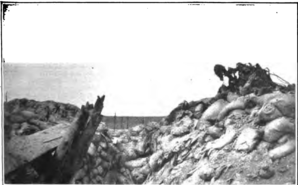
THE CONDITION OF THE DEFENSES ON HILL 304 AFTER A TERRIFIC BOMBARDMENT
